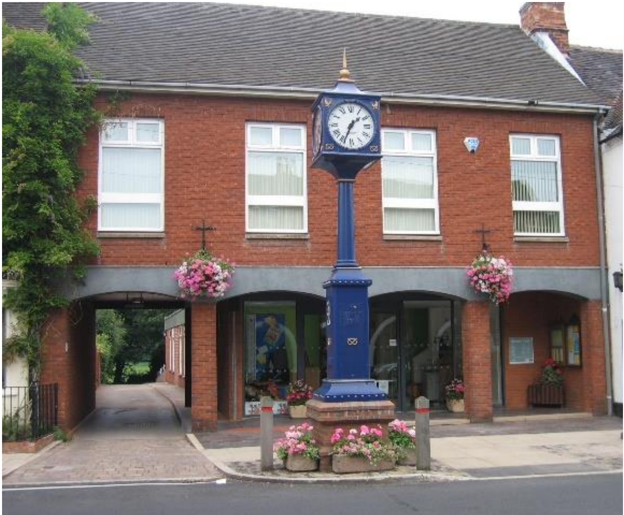
Eccleshall Library, High Street, Eccleshall
