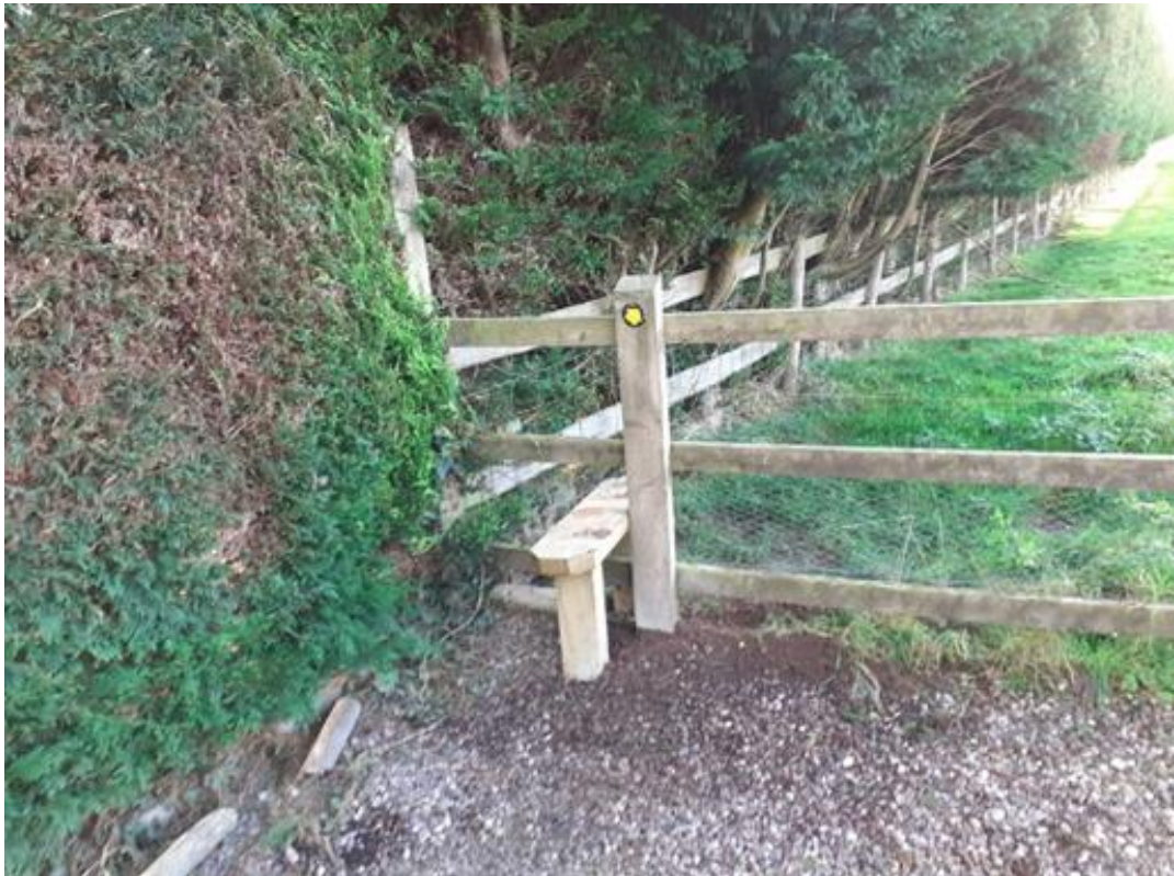
Parish Council footpath maintenance works to replace a stepper
